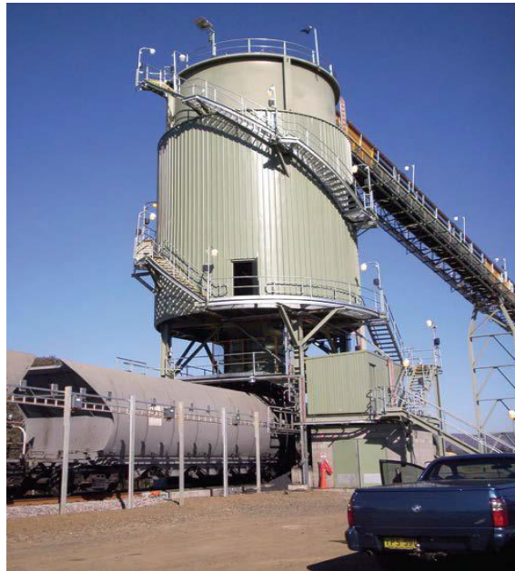
Figure 1.15 - Coal loading point (Australia) [89]
